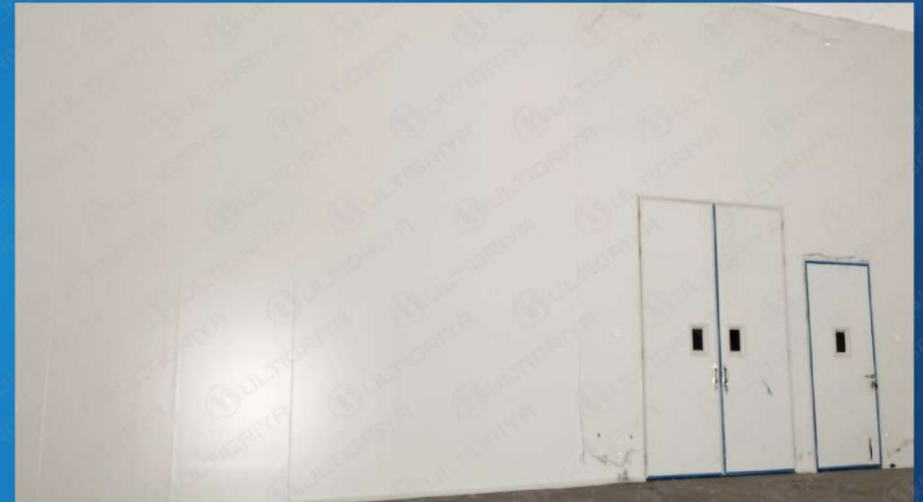
PT. CPMI, Banten Project Clean Room
