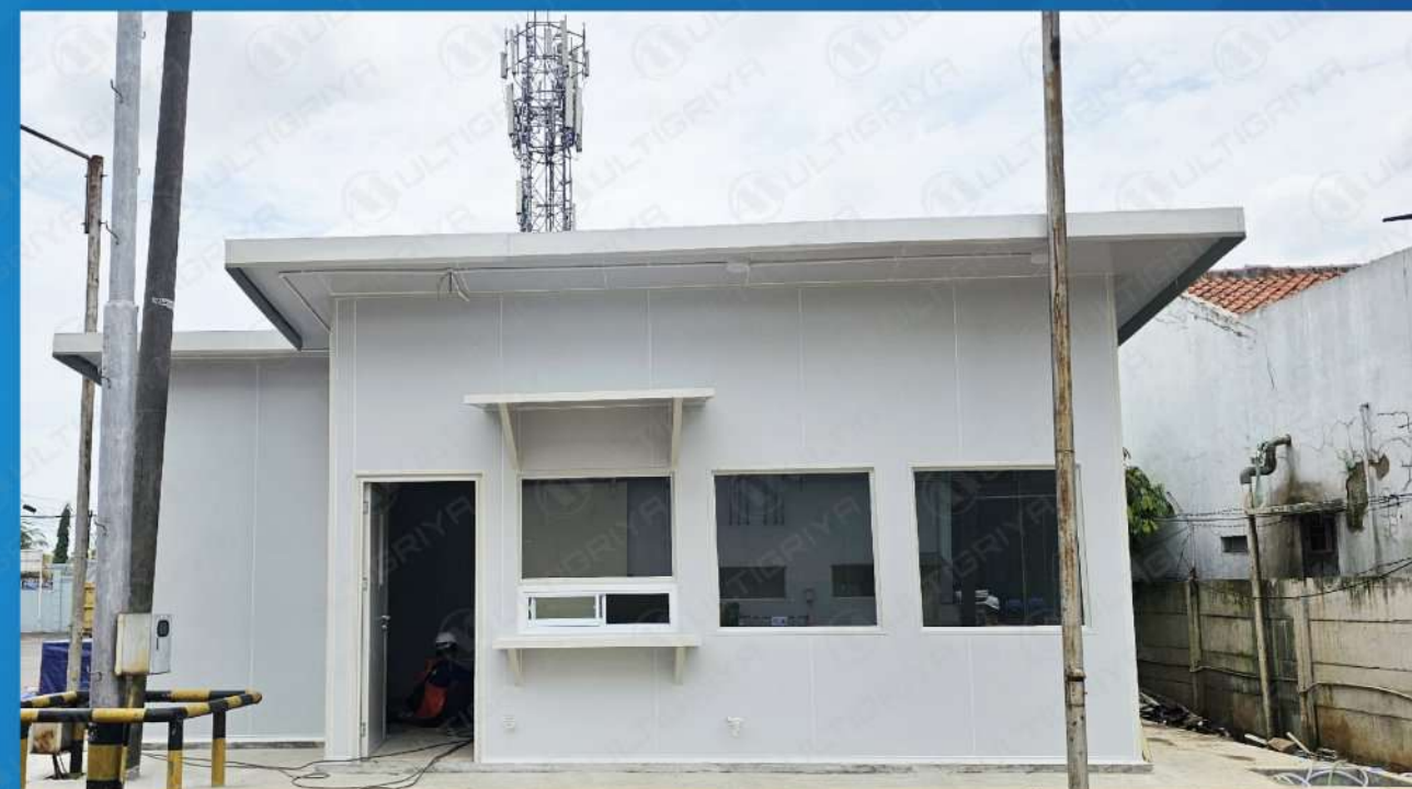
PT. BTM, Banten Project Operator Room
