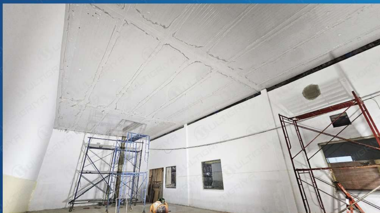
PT. SKR, Banten Project Clean Room Pabrik Makanan
