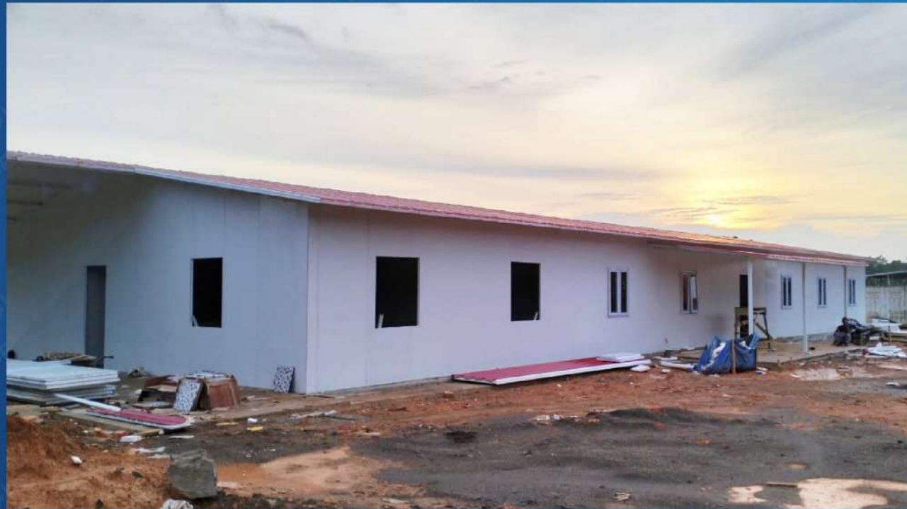
PT. DWP. Palembang Project Mess Karyawan
