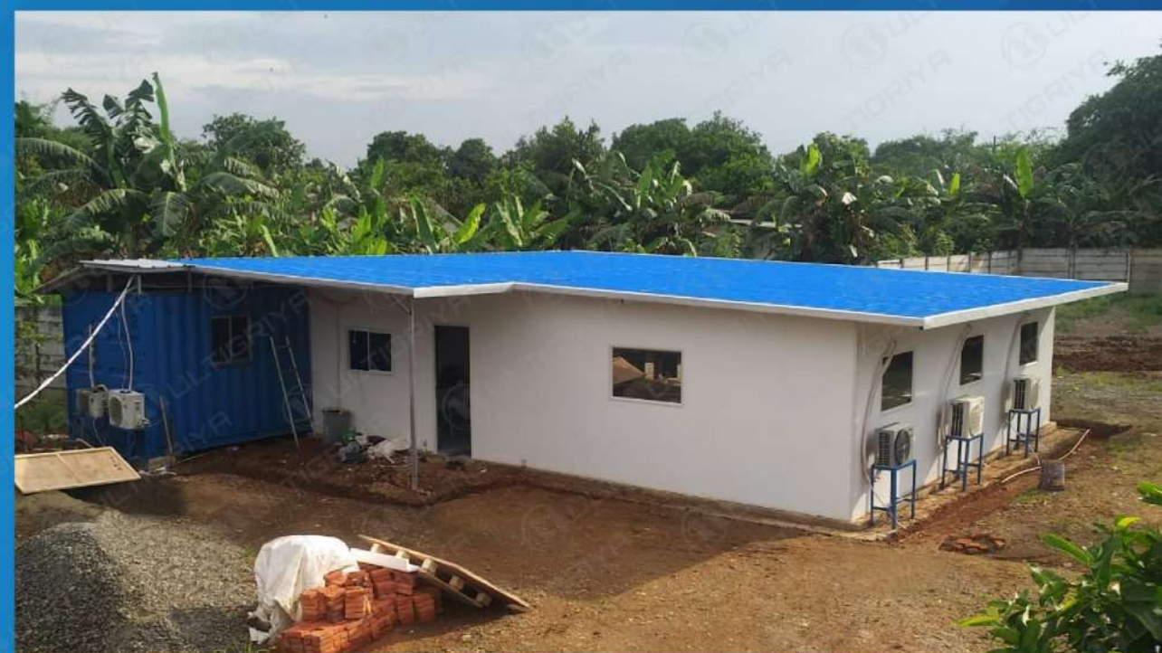
CV. IF, Banten Project Laboratorium
